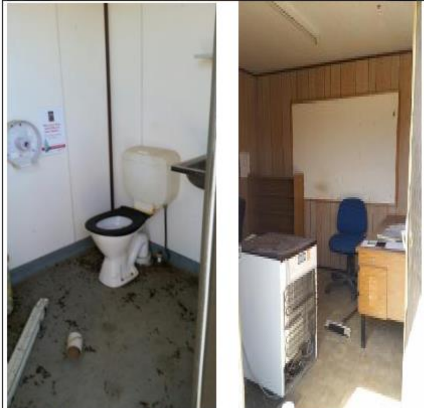
Toilet & office in existing demountable
