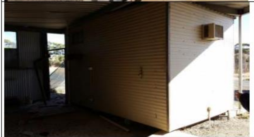
Existing demountable rear & side view
